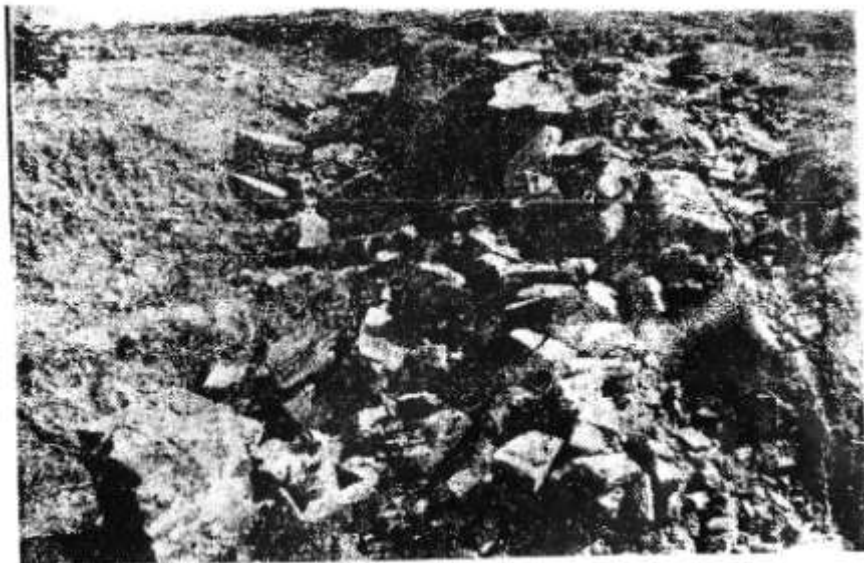
Boundary wall totally destroyed.
