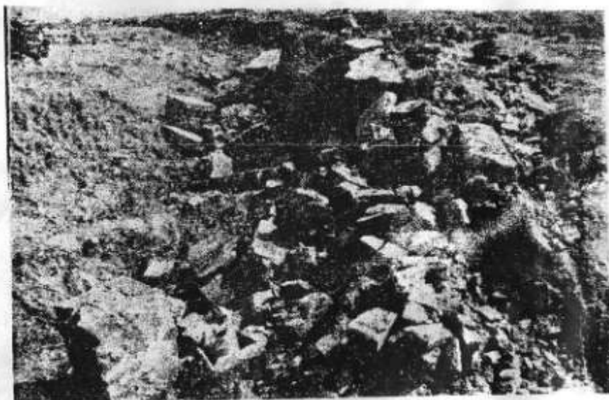
Boundary wall totally destroyed.
